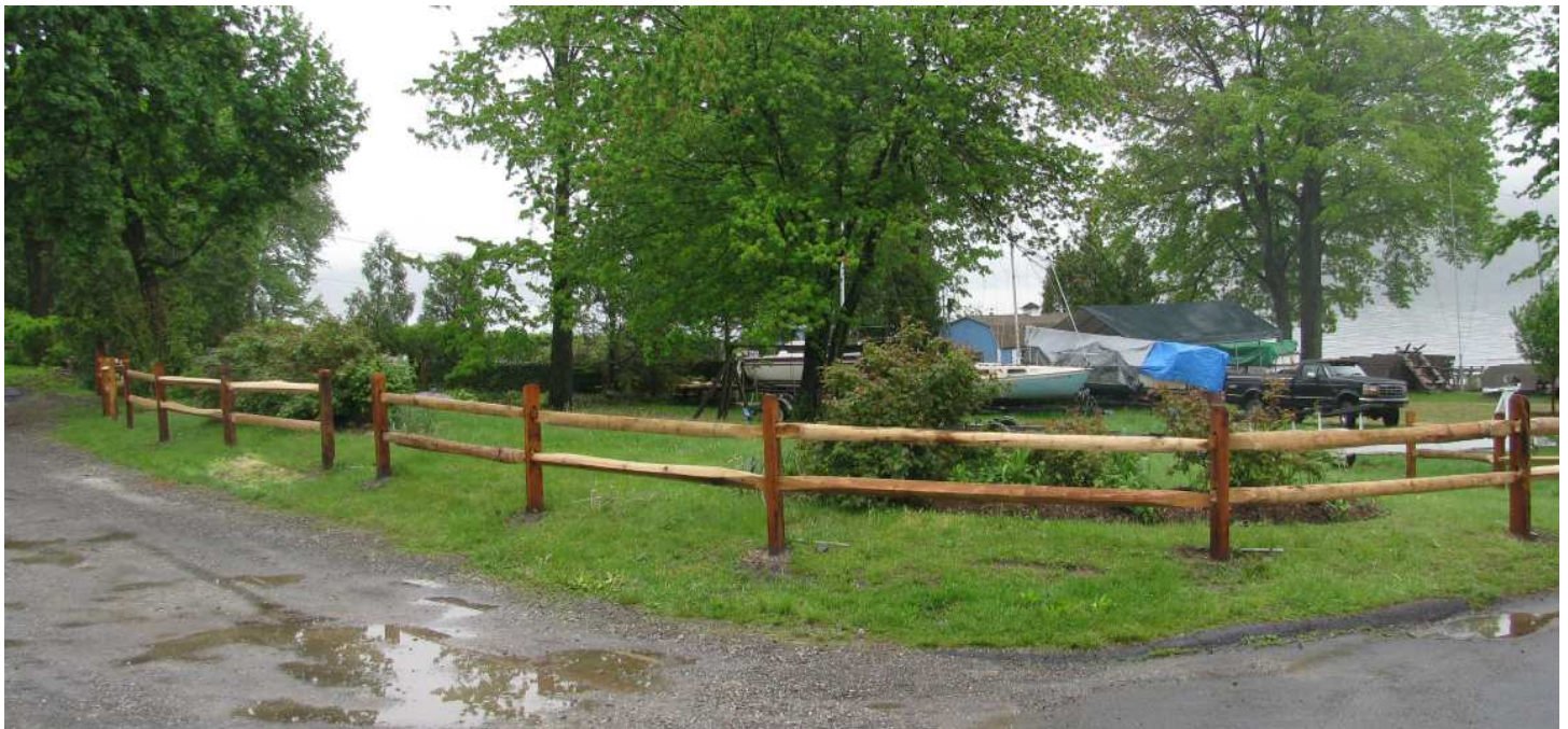
May 2011- the magnificent, new split rail fence
